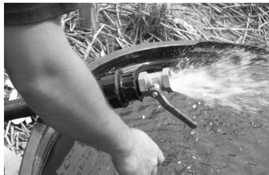
Figure 13.10 In order to increase the water pressure to Sungei Tekam village so that the whole village can be supplied, a 300 feet extension pipe was added in 2008. This served to raise the intake upstream to a higher point and thereby increase the water head.
